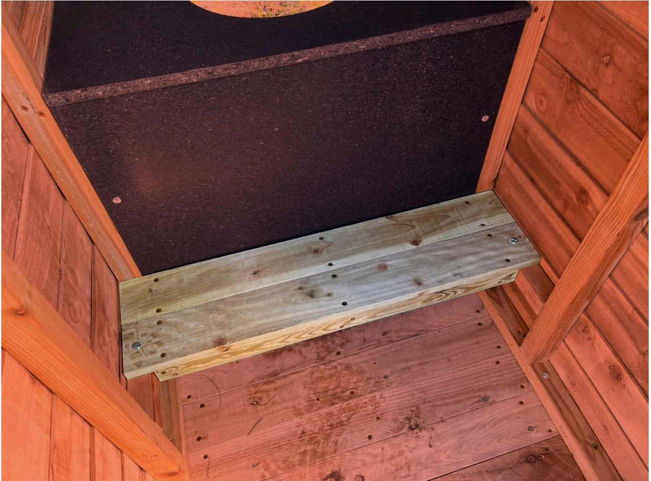
Secure in place using **two** 80mm bolts from the top, and secure with washers and nuts from below.
