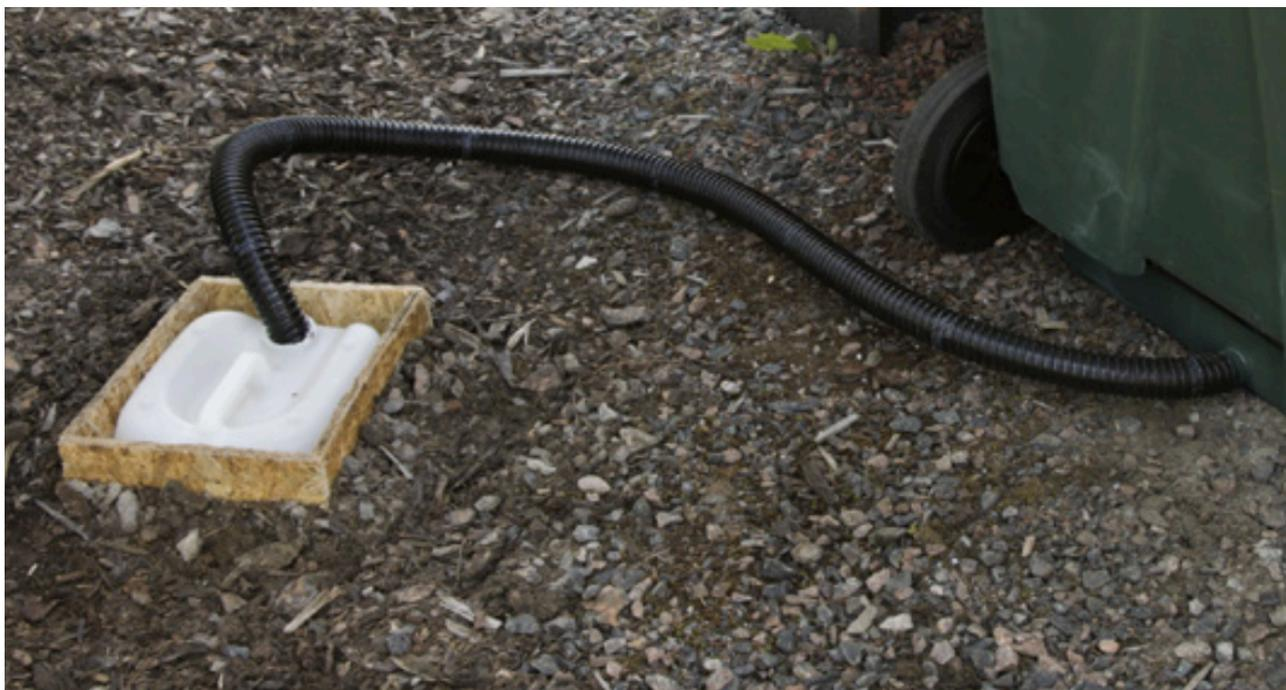
Run the leachate pipe into the top of the container and check the level regularly.
