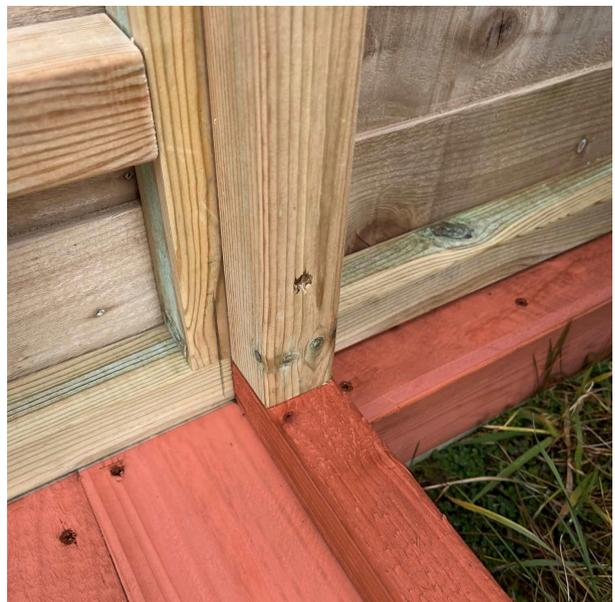
You will need someone to hold the side panel upright and steady as you insert **four** of the 80mm bolts into the holes.
