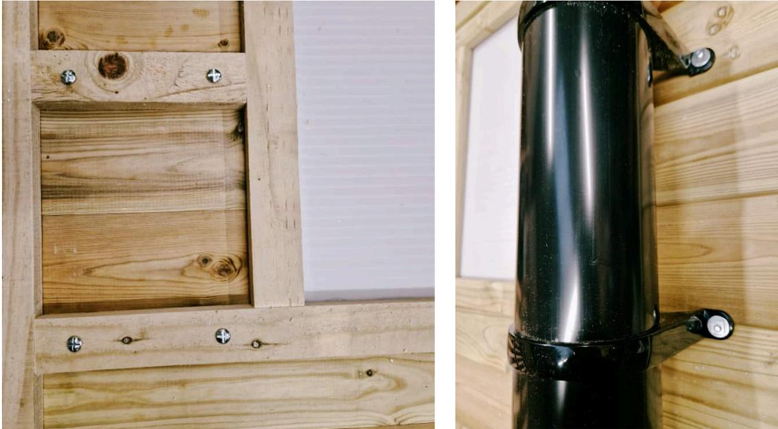
Fit the two support brackets on the pre-formed vent pipe. From the outside, offer the support brackets up to the protruding bolts and loosely secure with a washer and nut. It can be helpful to have someone inside the cabin to keep the bolts in place until the washer and nut is on.
